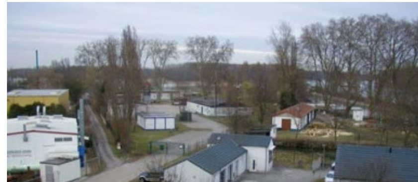
Buildings in the floodplain
